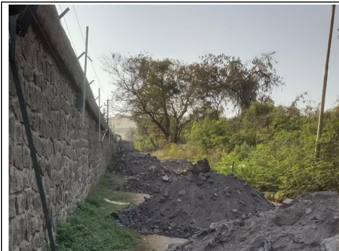
Construction of road using slag dump within the plant
