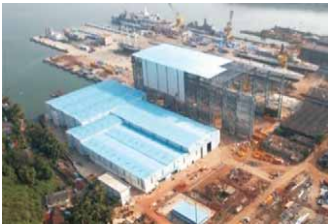
Ongoing Modernisation for MCMV Project
