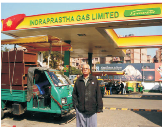
CNG Station operated by ESM(O) in NCR
