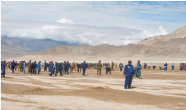
Air warriors clearing the runway from mud caused due to the landslides
